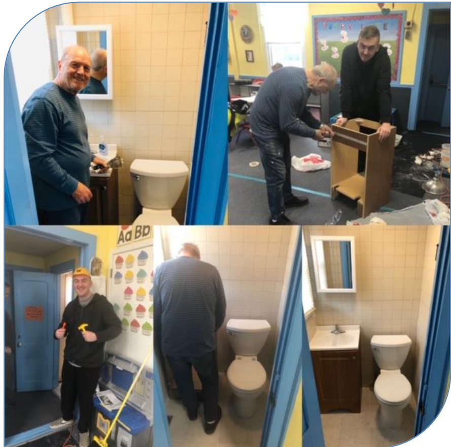
A new lavatory has been installed in Parish Hall!
