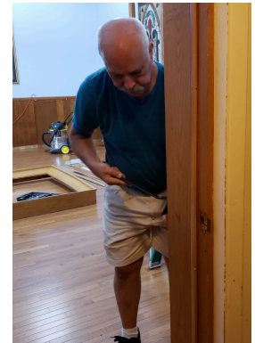
Rex Enderlin replacing door molding in the Chapel
