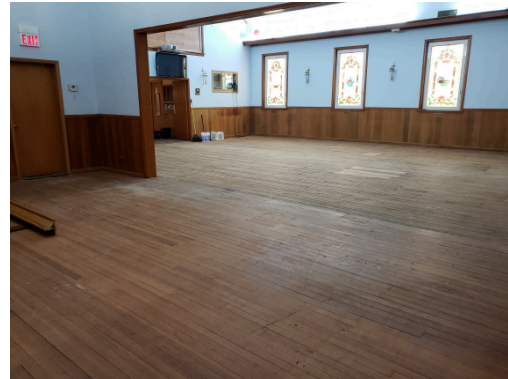
Original 1906 floor under carpet
